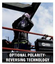
No cable swaps are needed, so switching processes is quick and simple.
